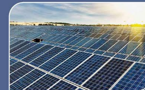
5000 MW POWER PLANT AND SOLAR PARK
