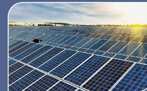
5000 MW POWER PLANT AND SOLAR PARK
