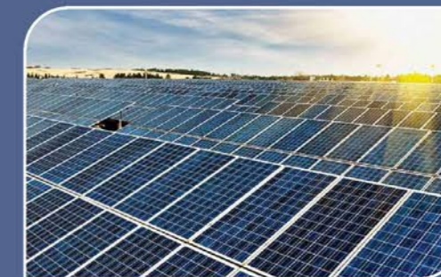
5000 MW POWER PLANT AND SOLAR PARK
