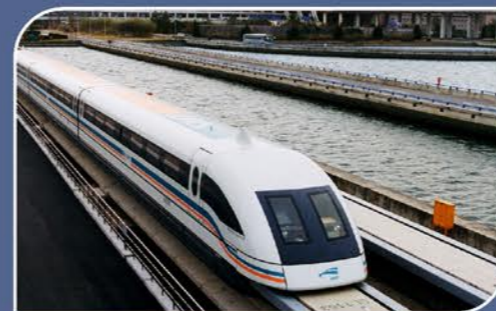
Metro Railway (Dholera to Gandhinagar Via Ahmedabad)
