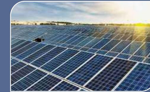
5000 MW POWER PLANT AND SOLAR PARK
