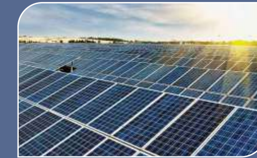
5000 MW POWER PLANT AND SOLAR PARK
